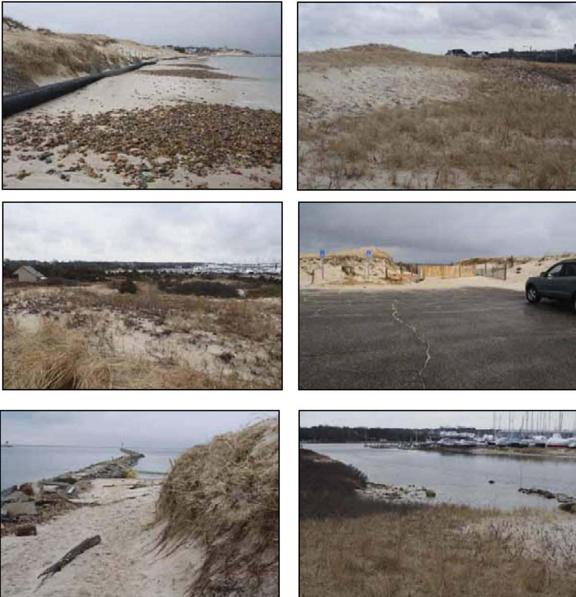
**Figure 4-8. View of Cold Storage Beach showing narrow beach with cobble covered cusps; wide, well vegetated coastal dunes; paved parking area; and Sesuit Harbor jetty with mid-section that has collapsed allowing erosion of the dunes (bottom right).**
