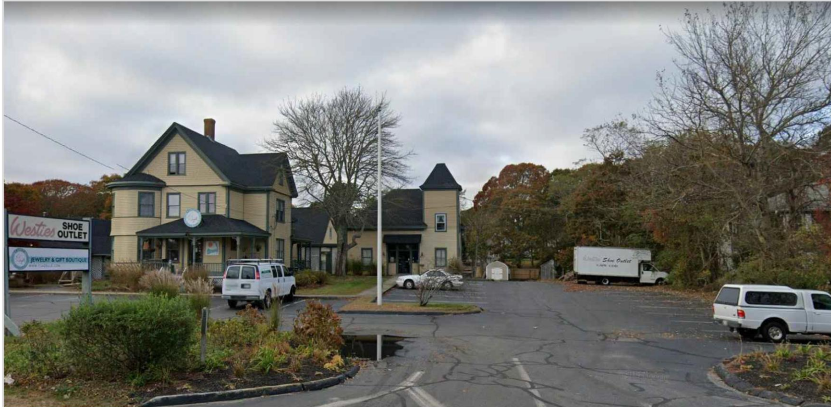
VIEW NORTHWEST FROM MASSACHUSETTS ROUTE 28/MAIN ST
