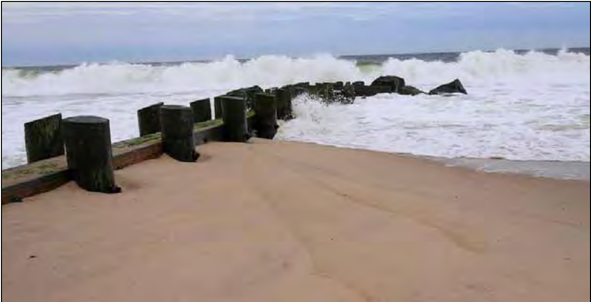
Figure 13: Example of Timber Groin, where Height cannot be Adjusted
