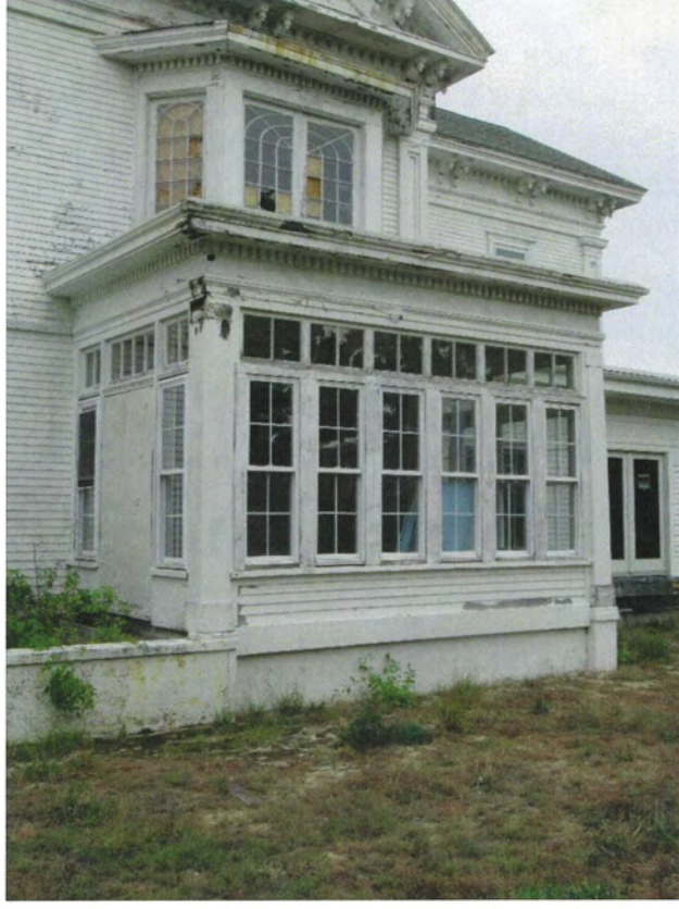
20. West elevation, sunporch, view southeast
