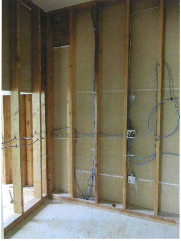
87. Second floor, northeast room closet, view southeast
