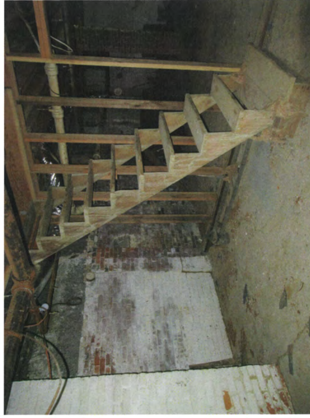
23. Basement stair, view southeast
