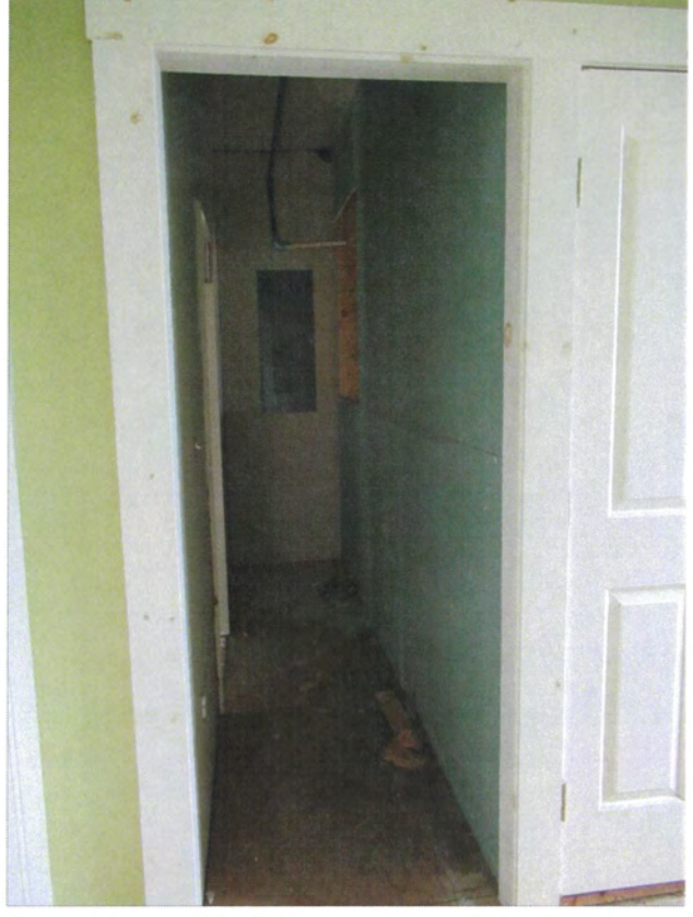
72. Second floor, rear stair hall corridor, view north
