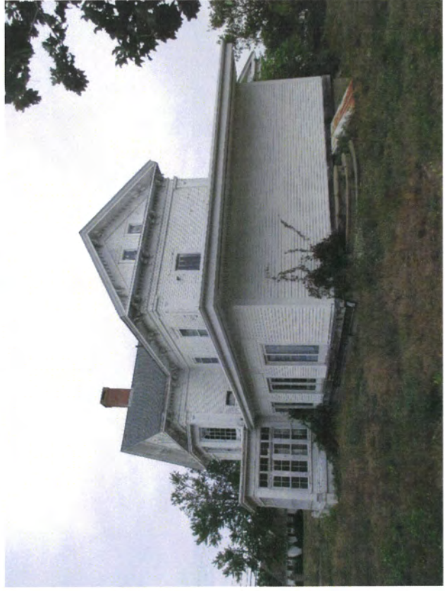
15. West elevation (left) and south elevation (right), with south addition in foreground, view northeast
