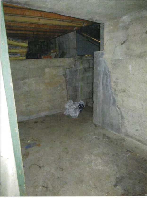
30. Basement, view southeast
