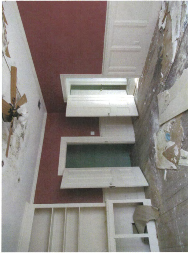
67. Second floor, southwest room, view southeast
