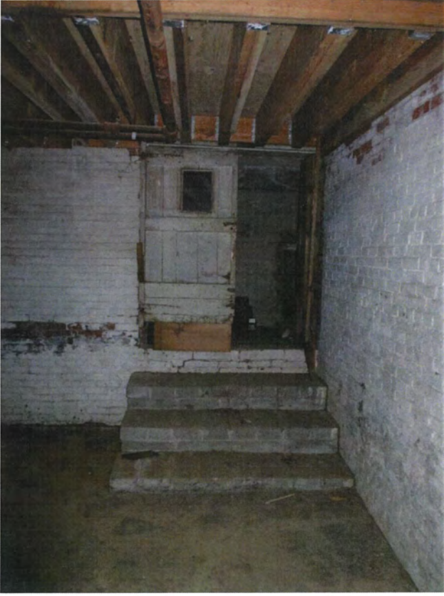
29. Basement, view south
