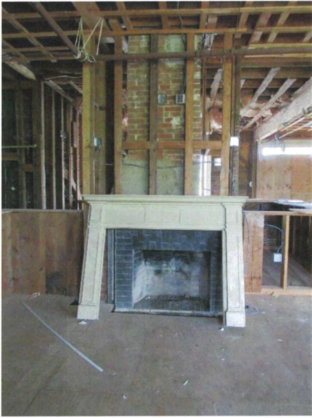
53. First floor, southeast room fireplace, view north
