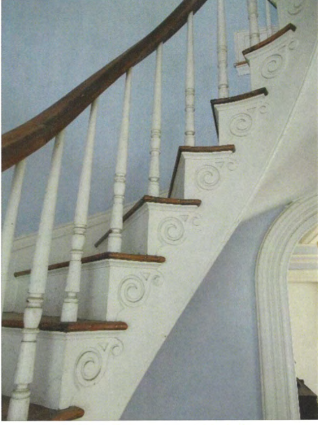
34. First floor, main stair detail, view southeast
