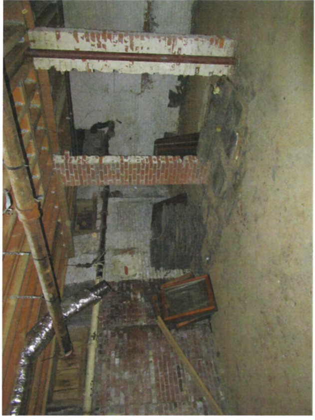
28. Basement, view southeast
