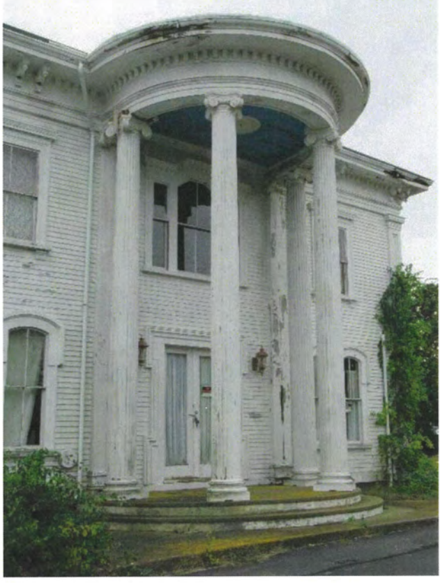
4. North elevation, portico, view southwest
