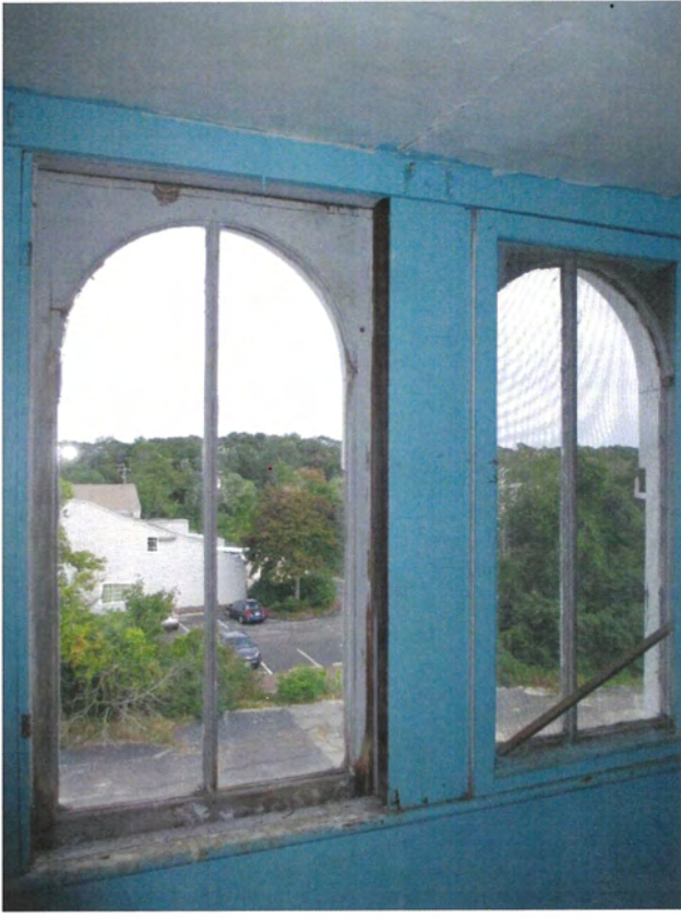
94. Third floor, east room window detail, view southeast
