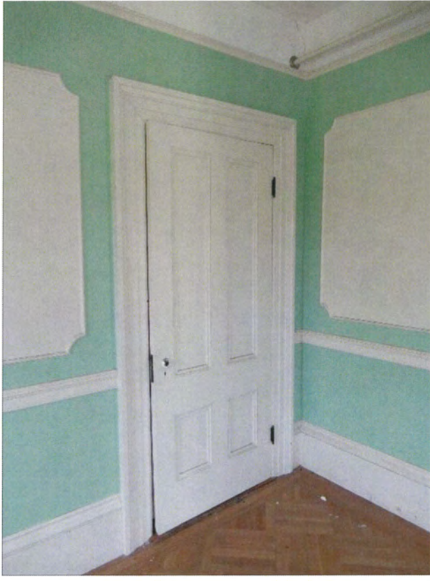
86. Second floor, northeast room, closet door, view southwest
