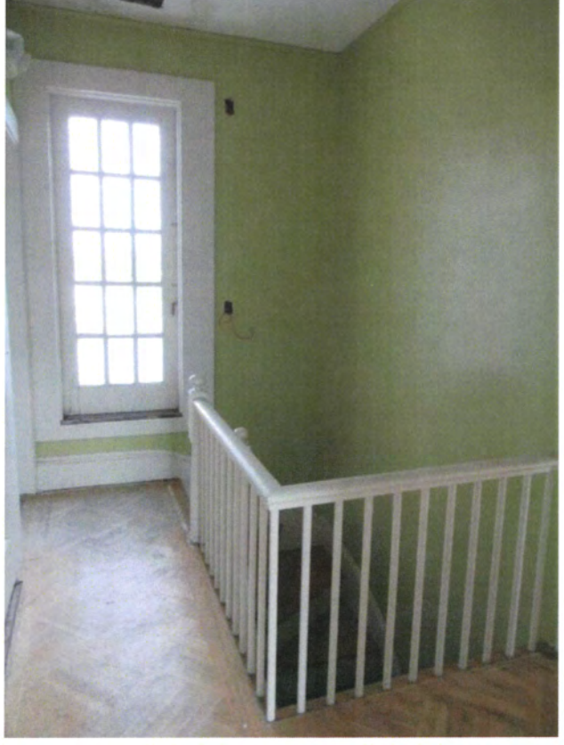
75. Second floor, rear ell stair hall, view east
