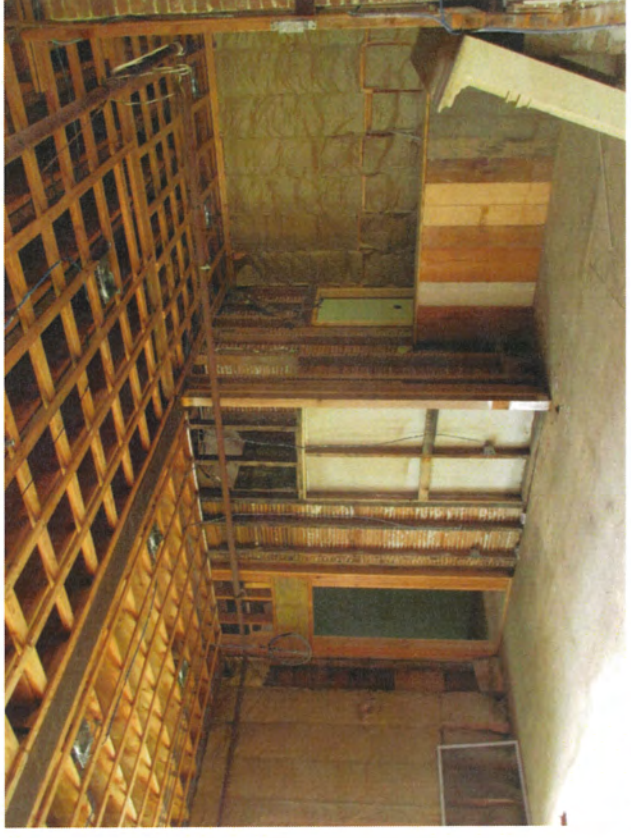
52. First floor, southeast room (right) and southeast addition (left), view southwest
