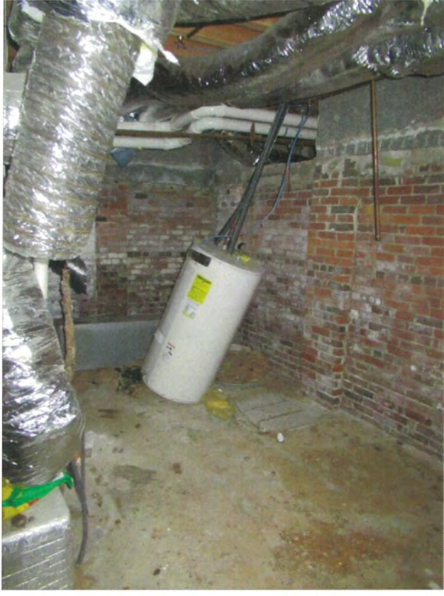
26. Basement, view east
