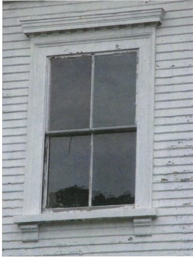
21. West elevation, second floor window, view east
