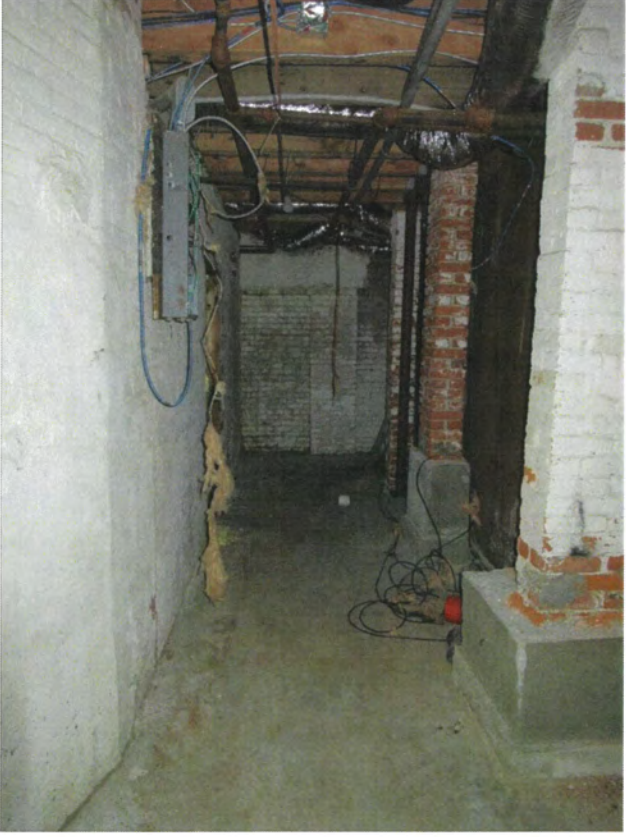
25. Basement, view north
