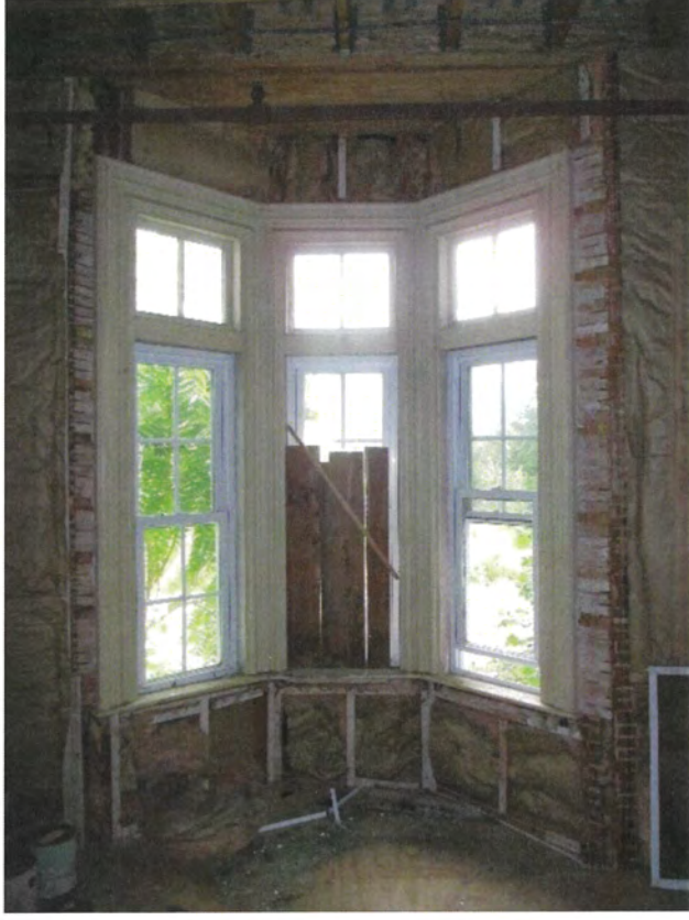
54. First floor, southeast addition window detail, view south
