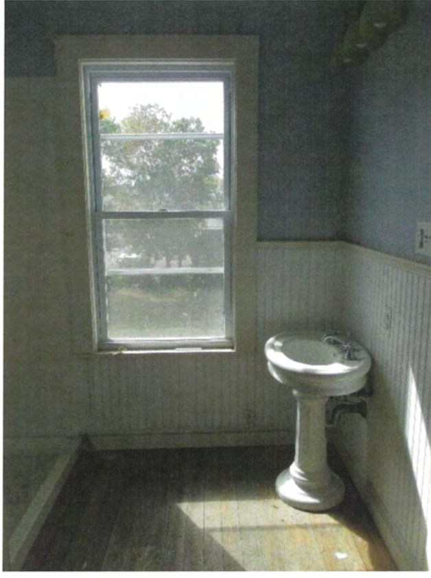
70. Second floor, rear ell bathroom, view west
