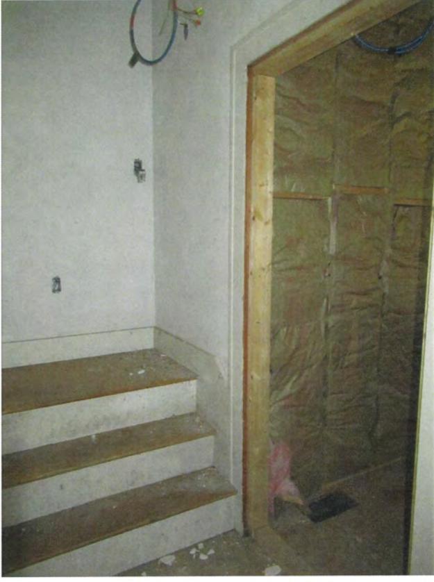
50. First floor, rear ell stair hall, view west
