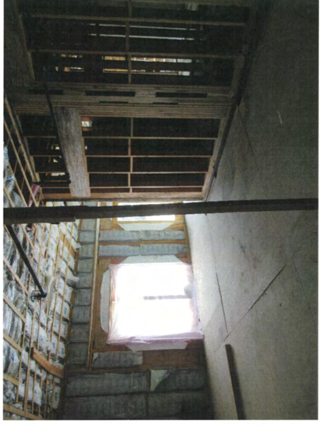
48. First floor, south addition and rear ell, view northwest
