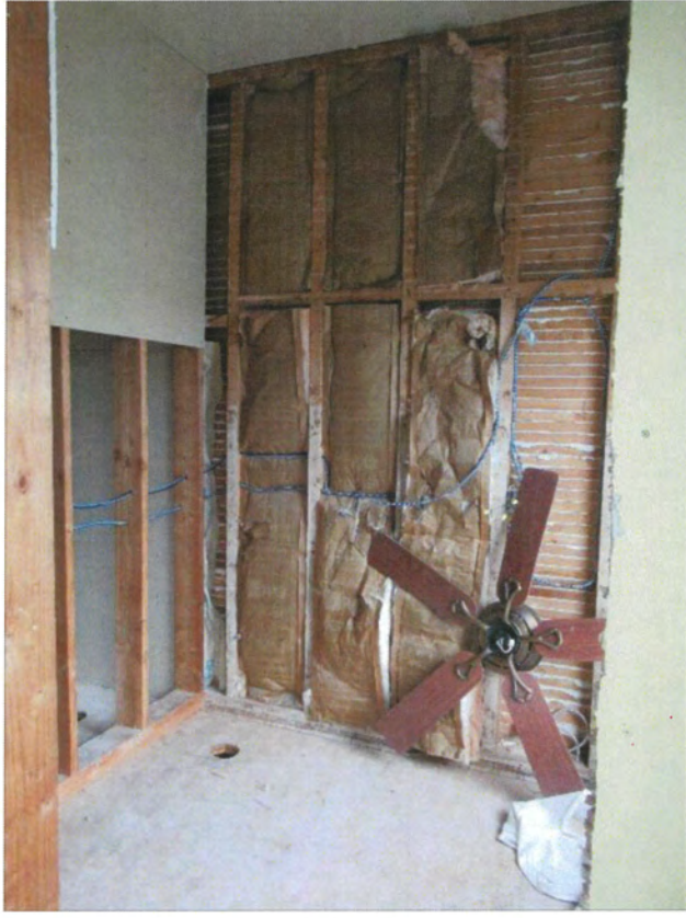
82. Second floor, southeast room closet, view northwest
