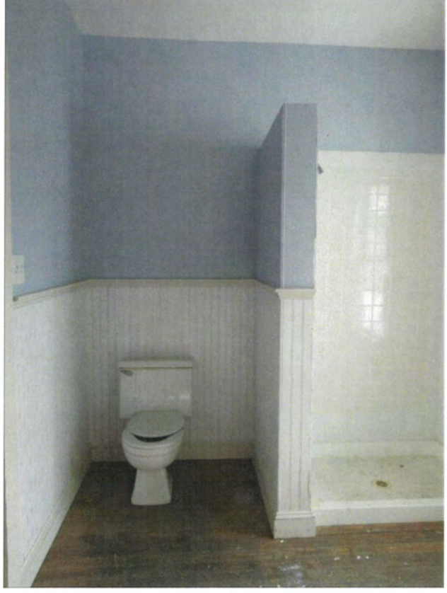
71. Second floor, rear ell bathroom, view south
