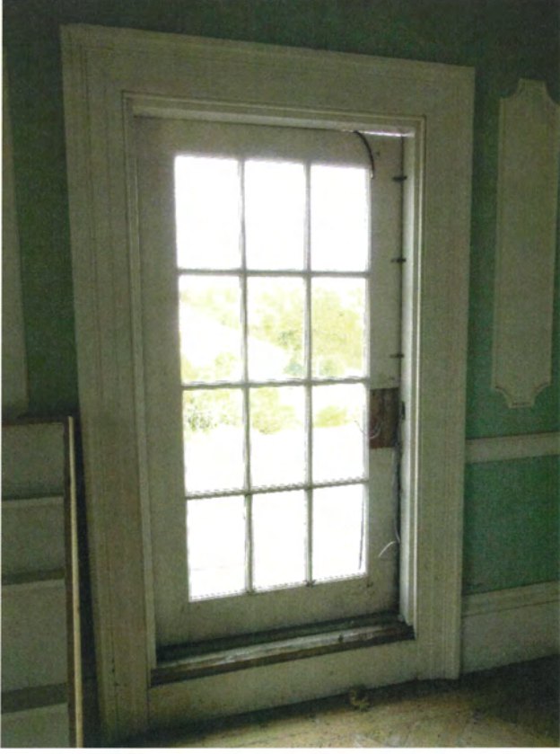
85. Second floor, northeast room, door detail, view east
