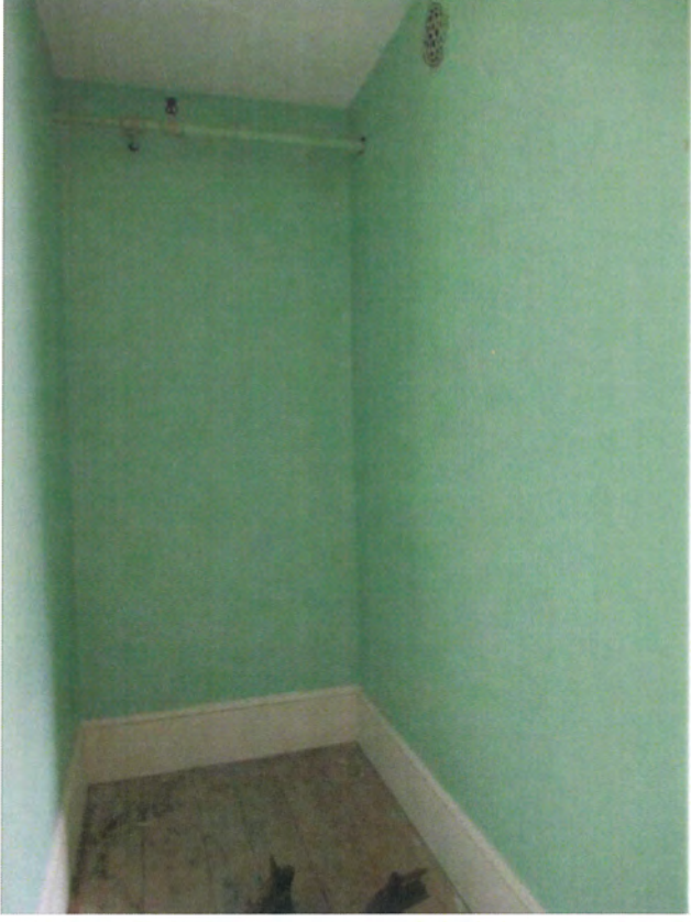
69. Second floor, southwest room closet, view east
