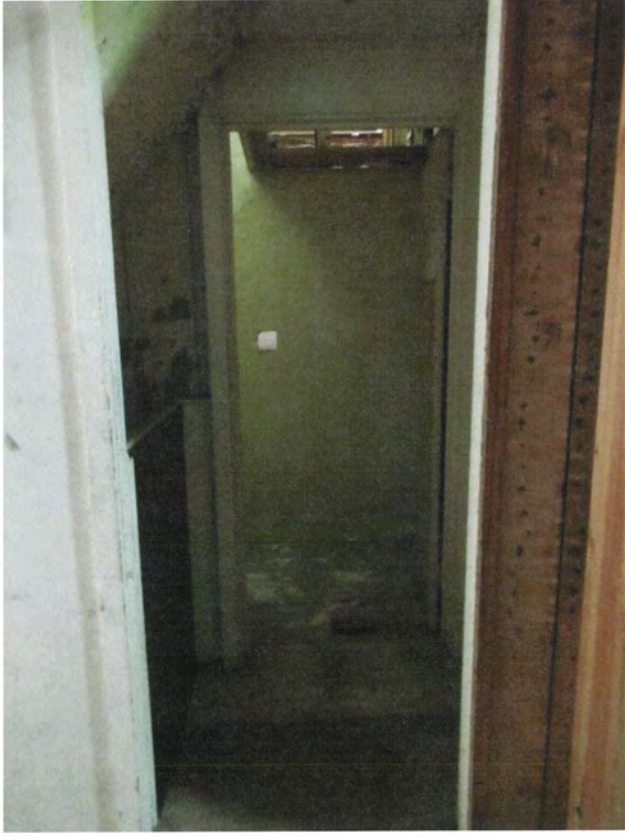
49. First floor, rear ell basement stair landing, view south
