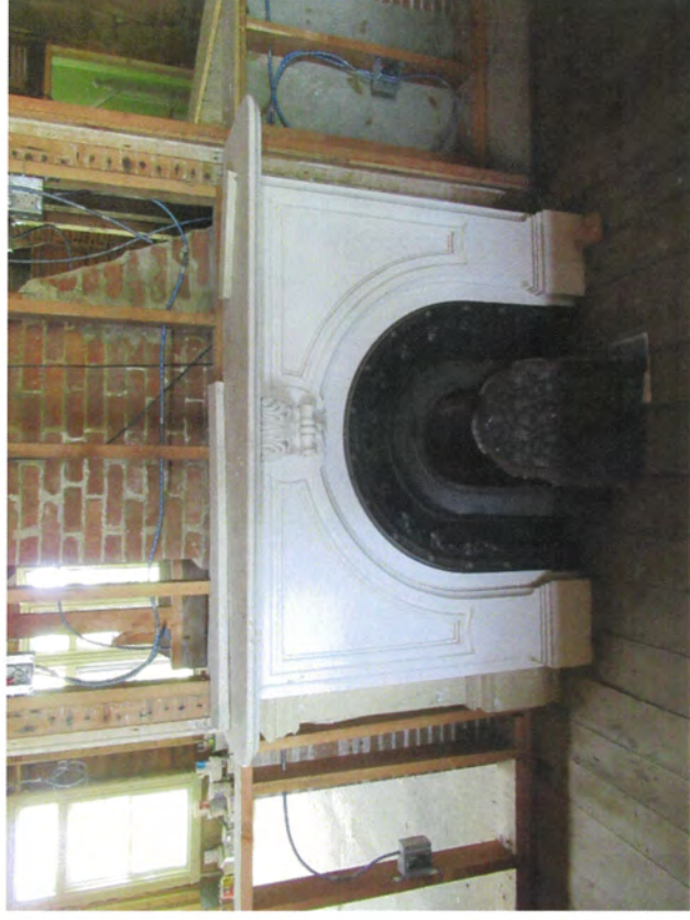
60. First floor, northeast room fireplace, view south
