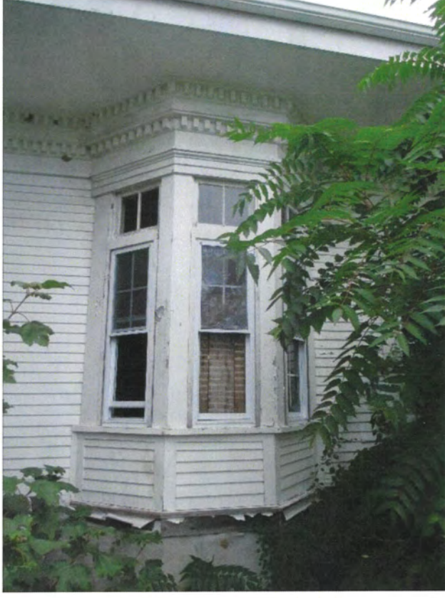
14. South elevation of southeast extension, window, view northeast
