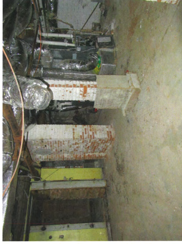
24. Basement, view northeast
